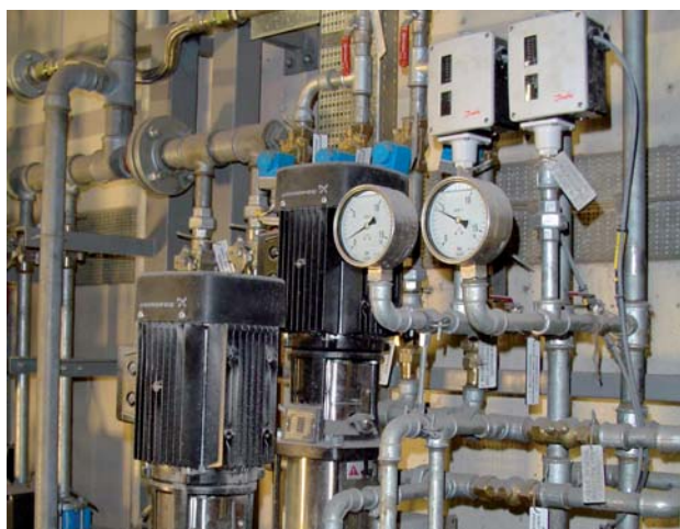
Two units on one skid supporting 2 boilers.
